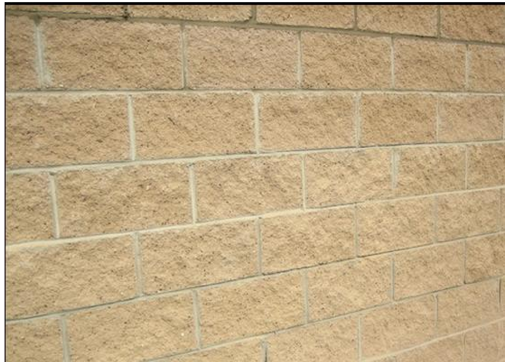
SPLIT FACE BLOCK WITH SPLIT FACE CAP- COLOR TO BE TAN- ORCO BLOCK OR SIMILAR
