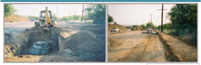
The Agua Mansa Road Improvement Project is a much needed improvement and widening of the Agua Mansa Road for future development. The project consists of preparing the road for widening by grading, trenching and placing pipe for new utilities. The quality control needs for this project relied heavily on the testing of the Recycled Rubberized Asphalt. Due to MTGL Inc.'s experience in this type of work, the Agua Mansa improvement has been another quality product.
