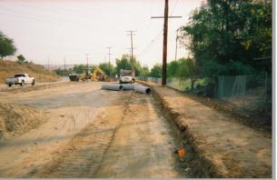
The Agua Mansa Road Improvement Project is a much needed improvement and widening of the Agua Mansa Road for future development. The project consists of preparing the road for widening by grading, trenching and placing pipe for new utilities. The quality control needs for this project relied heavily on the testing of the Recycled Rubberized Asphalt. Due to MTGL Inc.'s experience in this type of work, the Agua Mansa improvement has been another quality product.
